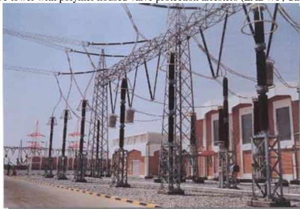
Figure 9:- Various Application- Toshiba 400kV surge arresters can be applied to extra heavy pollution area.
